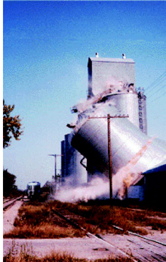
Figure 1.2: Industries handling granular materials often encounter problems of which this collapsing bin is a disastrous example... (from [6])
